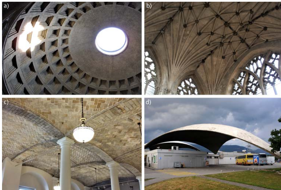
Figure 1 – Curved structures have been used to make use of brittle materials for millennia. Examples include a) the Roman Pantheon (completed 125AD), b) Ely Cathedral (1349), c) Boston Public Library (1895) and d) Heinz Isler’s Deitingen motorway service area (1968).
